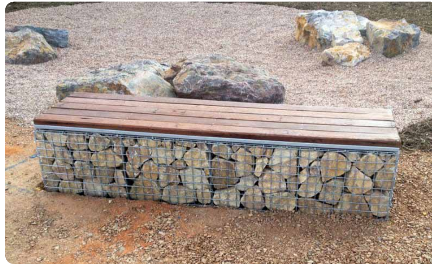
Gabion wall seating
