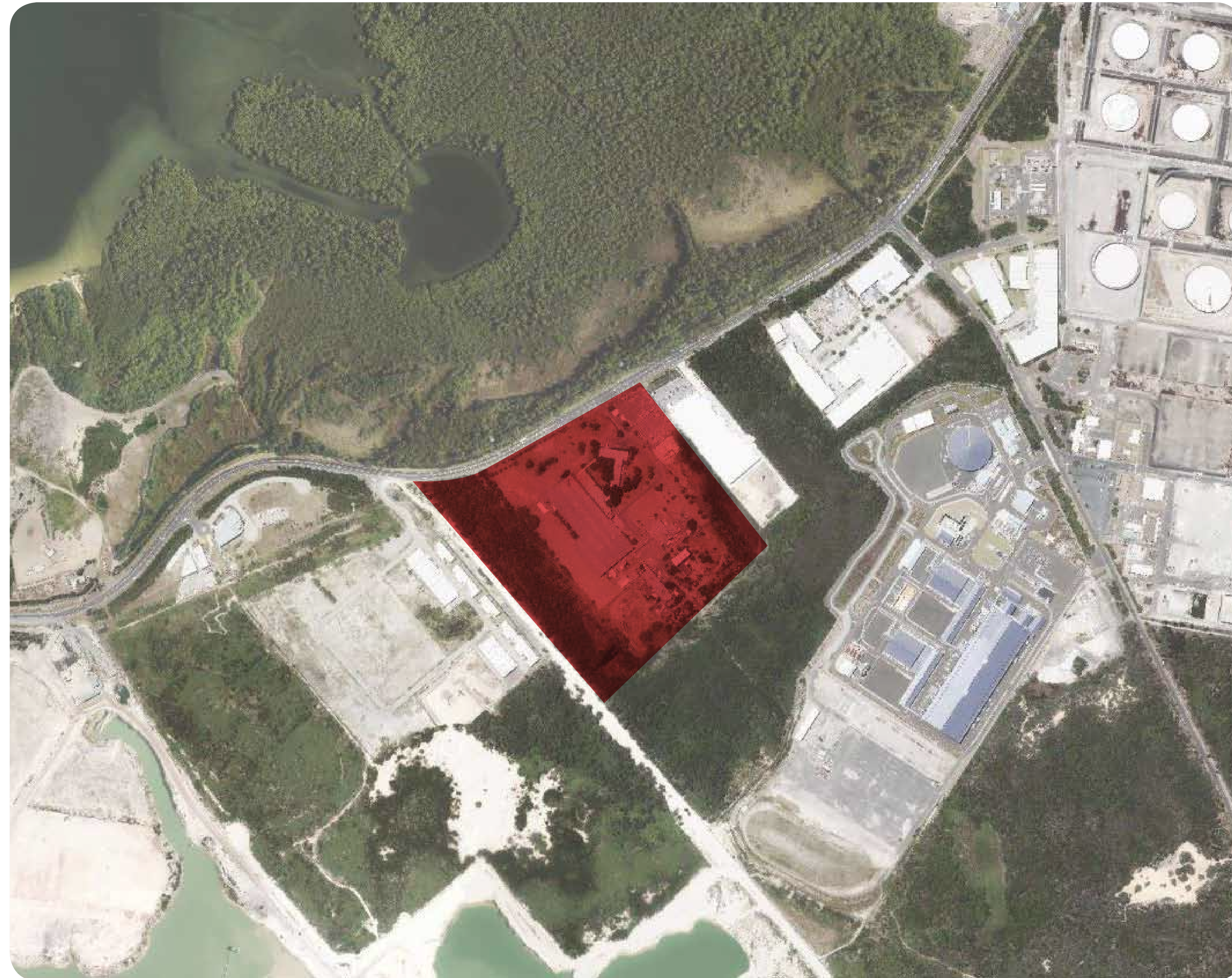
DICKER DATA OFFICE & WAREHOUSE DEVELOPMENT - CAPTAIN COOK DRIVE, KURNELL
